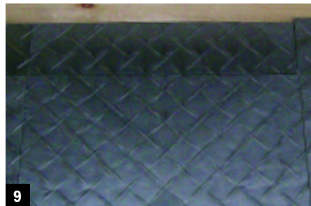
9 ...and popped the custom-cut tiles into place.
