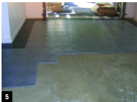
5 You should start in a corner and work from left to right and top to bottom, because of the way the tiles connect.
