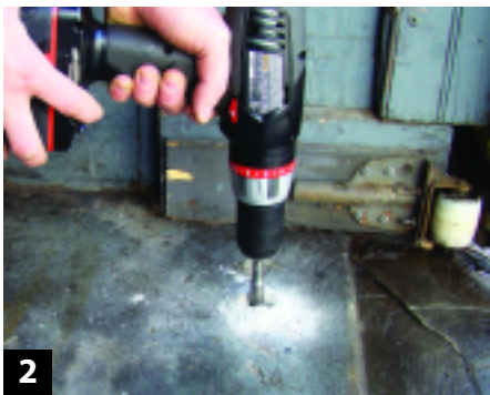
Select a location. The corner of a room will prevent a tripping hazard. Drill only one 5/8" hole at this time.
