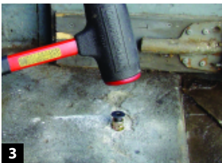
Remove the concrete dust with a vacuum or compressed air, and insert one Allen bolt and shield.
