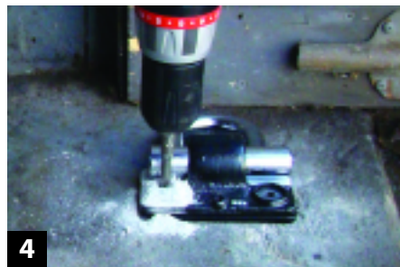
Place the T-base over the first mounting hole and bolt it down. Drill a 5/16" pilot hole for the second bolt point, and remove the T-base. Enlarge the second hole to 5/8", remove dust, and install the second bolt shield. Then continue the same procedure for the final hole.
